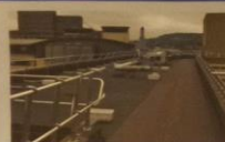
Experiment location (roof of the School of Applied Sciences, University of Huddersfield)
